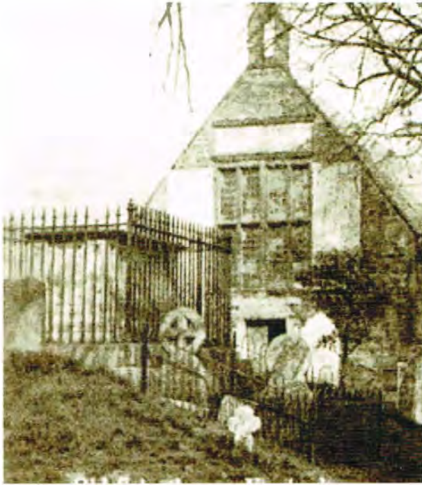
A casualty: these railings no longer exist
