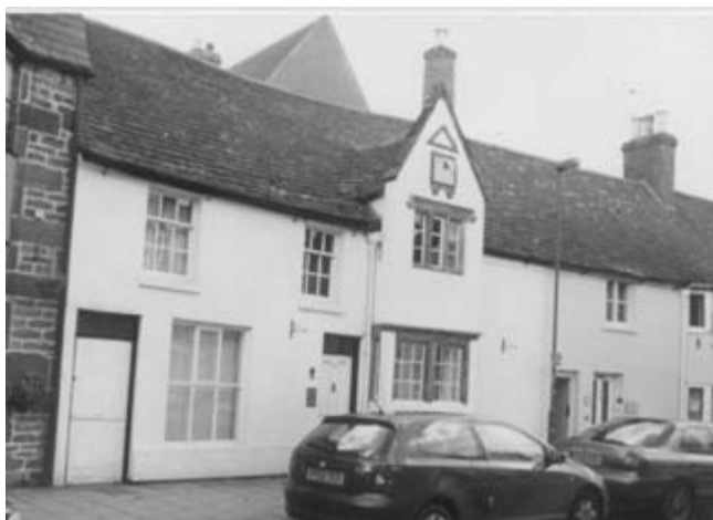
Fig 18a: 45 High Street East, a late medieval open hall and cross wing house of a type well known in the area.
