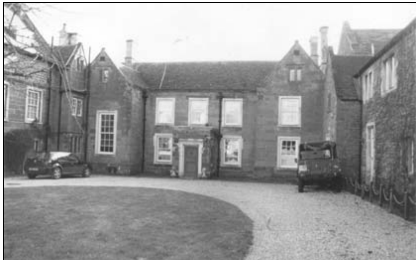
Fig 26: the Hall; a hall with two cross wings. A date stone says 1612 but it abuts against slightly earlier buildings; it has been refronted in the eighteenth century.
