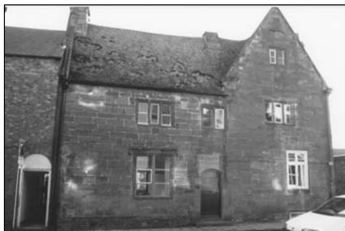
Fig 27: 50-52 High Street East, dated 1616; originally one house, it incorporates some medieval fragments. Smaller than Tudor House, it is however on much the same plan, hall with cross wing. The main entrance was almost certainly formerly at the rear.
