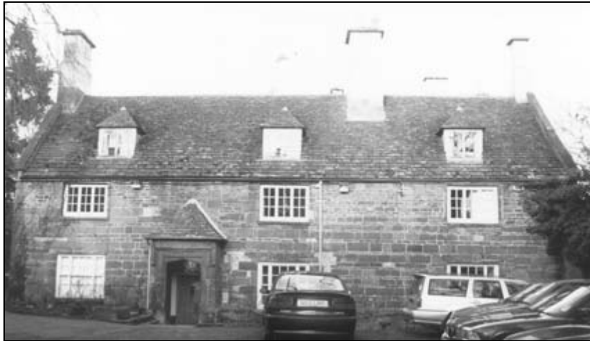
Fig 24: now called the Thring Centre, it is a late sixteenth or early seventeenth century building which needs detailed examination. The small windows indicate its early date (probably originally stone mullion windows); the porch is later. Who built it on such a grand scale?
