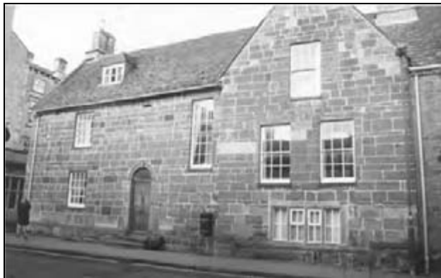
Fig 25: Tudor House, built on a traditional hall and cross wing pattern but on a massive scale (the original front door was at the rear); again note the different floor levels. In what way is it related to what is now the Thring Centre nearby?
