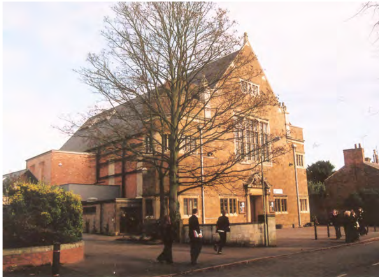
Uppingham Theatre and No 28 Stockerston Road
