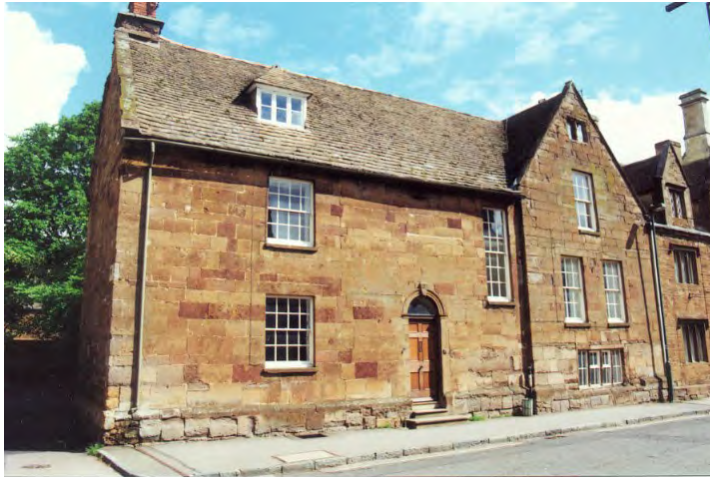
Tudor House 1, No 8 High Street West
